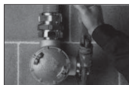
5. Install hub on enclosure
